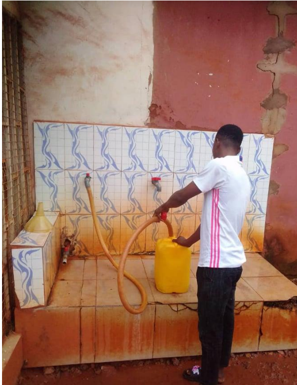
Figure 3: Resident collecting water from water point with a gallon
